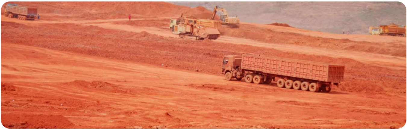
Heavy logistics — moving machines to the sites.
